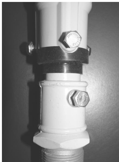
Figure 3: Figure 3 Installed Insect Boot
